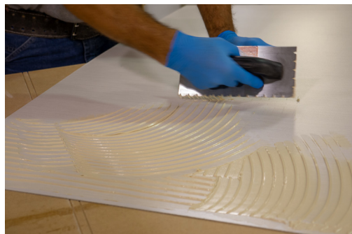
Apply adhesive. 100% adhesive coverage required.
