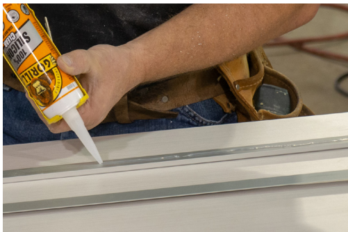
Use 100% clear silicone to adhere trim
