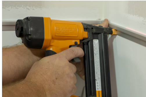
16-18 gauge 1" nails used to hold trim
